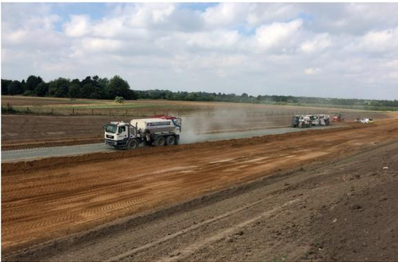
**1:** Spread TerraCem in a predetermined concentration on the surface.
