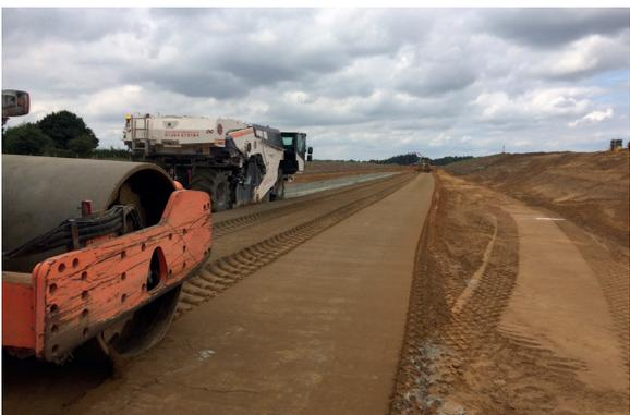
**5:** Complete the final grading and rolling with a steel drum roller.
