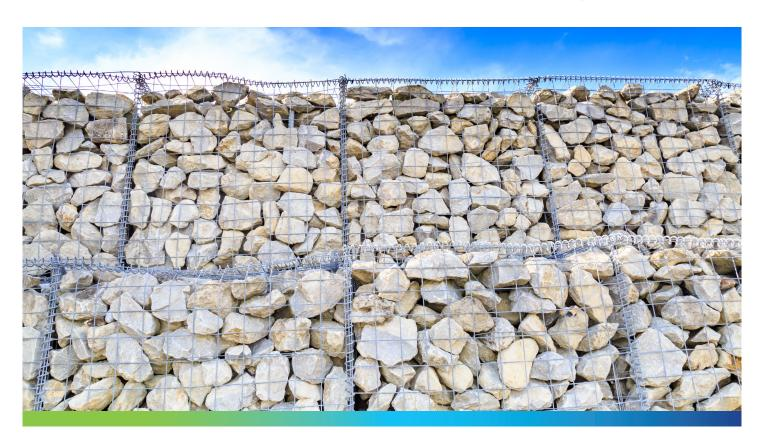
Gabion stone is a robust and versatile material used extensively in construction and landscaping projects. Known for its strength, durability, and aesthetic appeal, it is a popular choice for creating retaining walls, riverbank reinforcements, and decorative landscaping features. Whether used in infrastructure projects or garden designs, gabion stone combines functionality with environmental sustainability.
