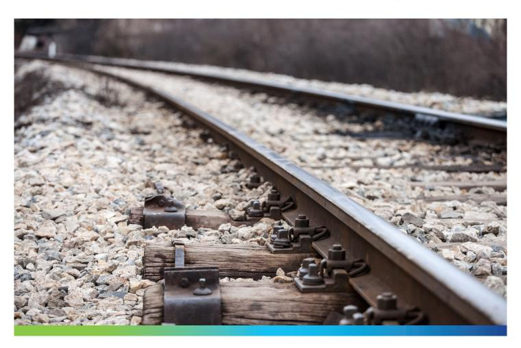
Rail Ballast produced from a number of aggregate types including crushed rock, recycled spent ballast forms the trackbed which serves as a solid bedding beneath railway tracks in order to ensure the smooth functioning of all railway systems. Holcim UK hard-wearing ballast acts as a level of protection for railway sleepers (railroad ties) in order to keep them in place and maintain optimal track alignment by packing between, below, and around the sleepers.
