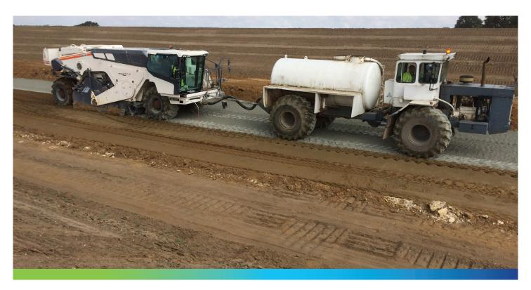
Designed to strengthen existing onsite material without the need to import aggregates, TerraCem soil stabiliser has been specially engineered to modify and improve soils, strengthening weak substructure layers to create a more robust working platform.
